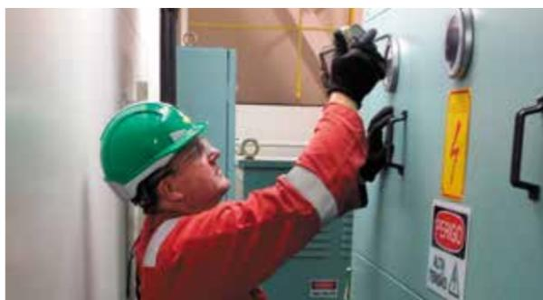
In servicing Pacific Drilling's fleet of high-specification, ultra-deepwater drillships, Geo Therm Ltd's professional installation service teams retrofit the CorDEX IW range of infrared window orders. This helps towards the performance of the annual offshore electrical thermographic survey inspections on the various rig-wide switchboards and HV transformers.
